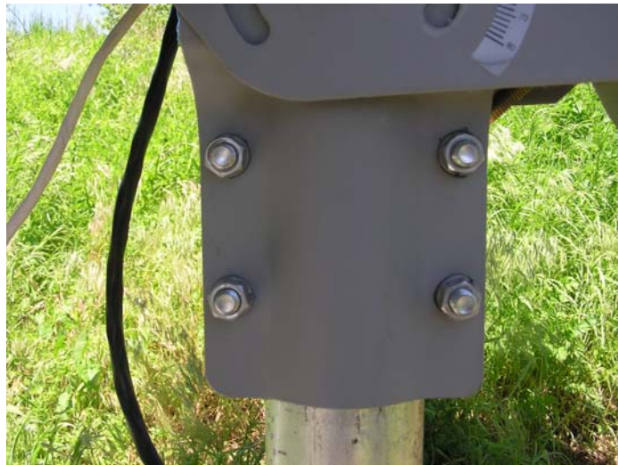
Figure 23 – Loosen Mount Clamp Bolts to Adjust East-West Bearing Angle
